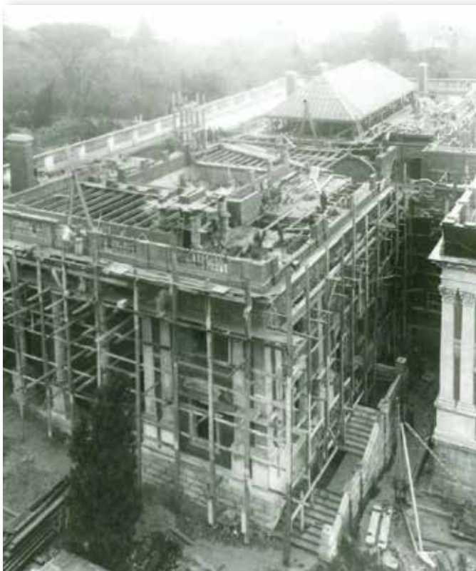
Construction work on Houses of Parliament in Cape Town
