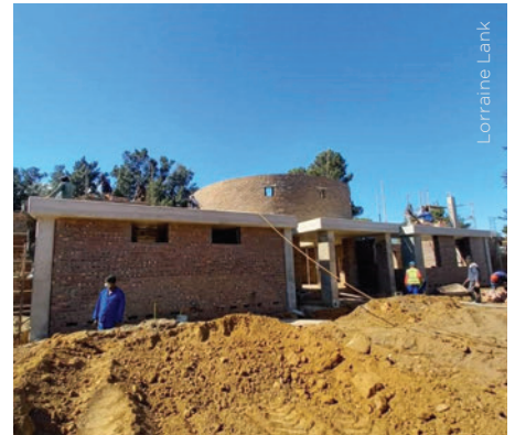
Construction of the Archbishop Desmond Tutu Public Library
