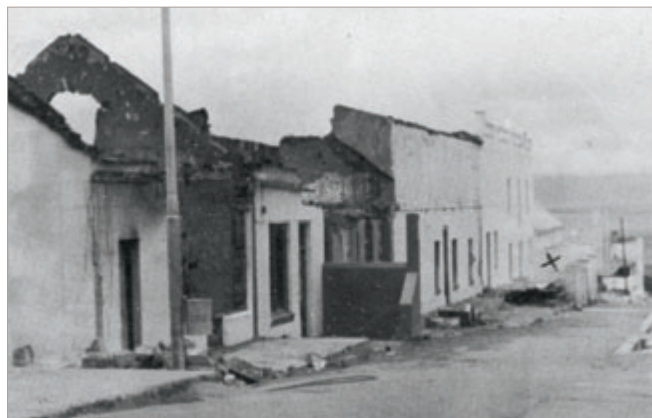
The scene of the fire at Piketberg Public Library in 1967
