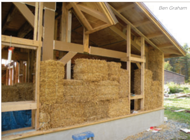
Construction of a strawbale home
