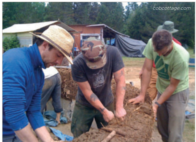
Building a cob cottage from earth mixed with sand and straw
