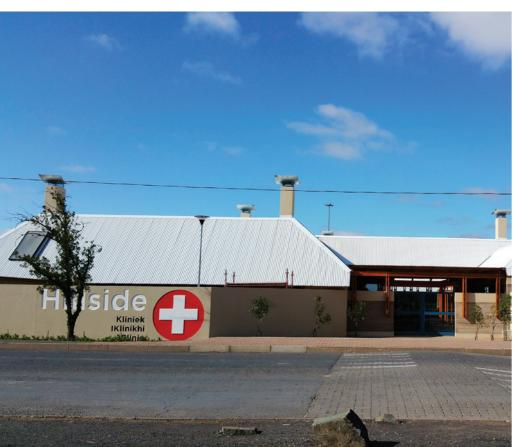
The new Hillside Clinic in Beaufort West contains the most "green" features facility in the Western Cape. Rammed earth walls and underground rock stores reduce the need for air conditioning by mitigating temperature extremes (high temperatures during the day, and cold temperatures at night). The design also features optimised natural daylight, energy-efficient heating, and a borehole for irrigating the water-wise garden.
