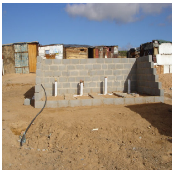
Construction of toilet facilities, Cederberg Municipality
