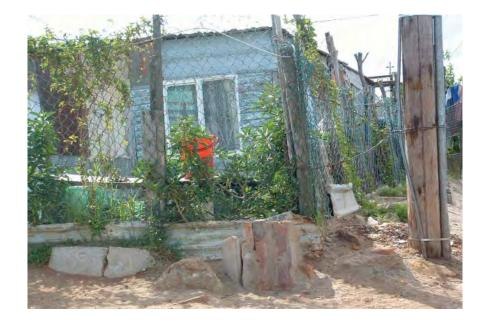
Zinc sheeting and concrete blocks laid around the plot to form a retaining wall, to prevent water flowing in from the road
