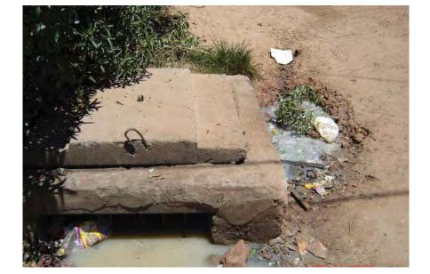
Over-burdened and blocked drains result in contaminated standing water
