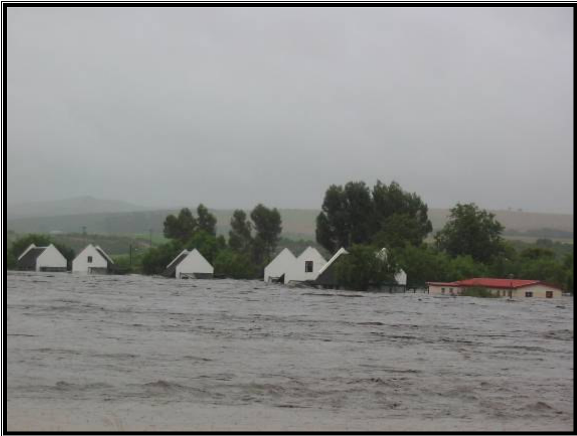
Fig 23: The Duiwenhoks River flooding the chalets in the Heidelberg Municipal Holiday Resort on the 22 nd December 2004.
