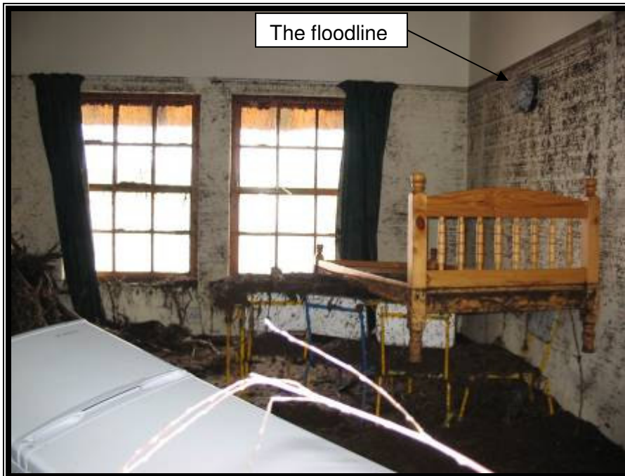
Fig 19: The interior of one of the Municipal chalets on the banks of the Duiwenhoks River. Photograph taken on the 23 rd December 2004.
