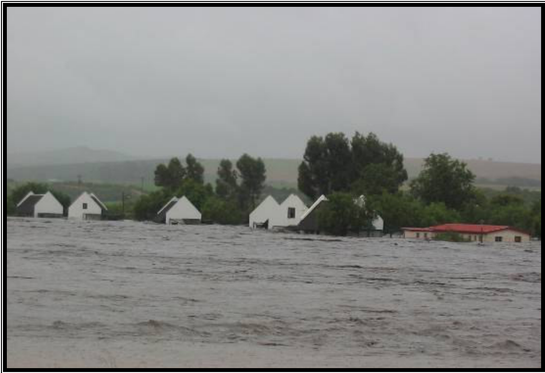
Fig 15: The Heidelberg Municipal chalets flooded by the Duiwenhoks River, 22 December 2004.
