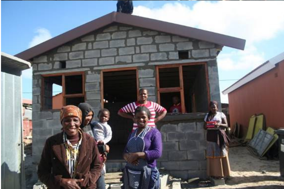
The completed home of Nolizwe Ntibane handed over just five days later.
