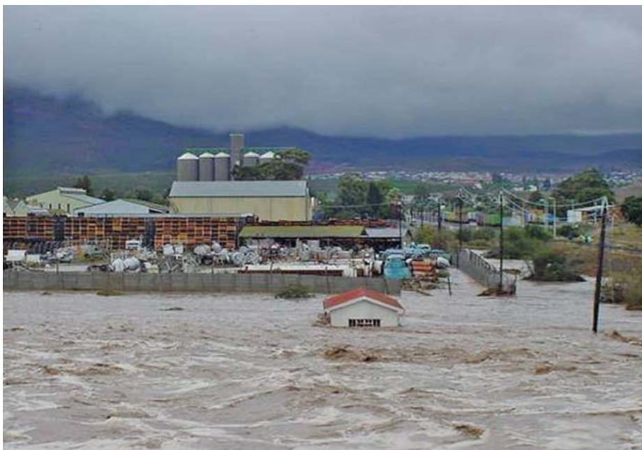
This image shows severe flooding in Ashton following the March 2003 'Montagu floods'. This event was not only reflected in serious damage to public infrastructure and agriculture. It also disrupted local livelihoods due to damage sustained by the local canning factories.
