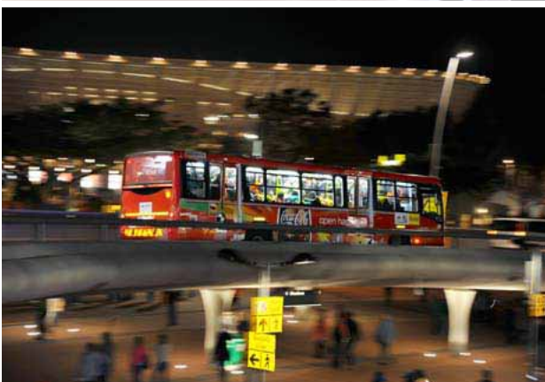
Pedestrian bridges, a new IRT system and a revamped Cape Town Station are legacies of the World Cup. Photos: Bruce Sutherland, City of Cape Town
