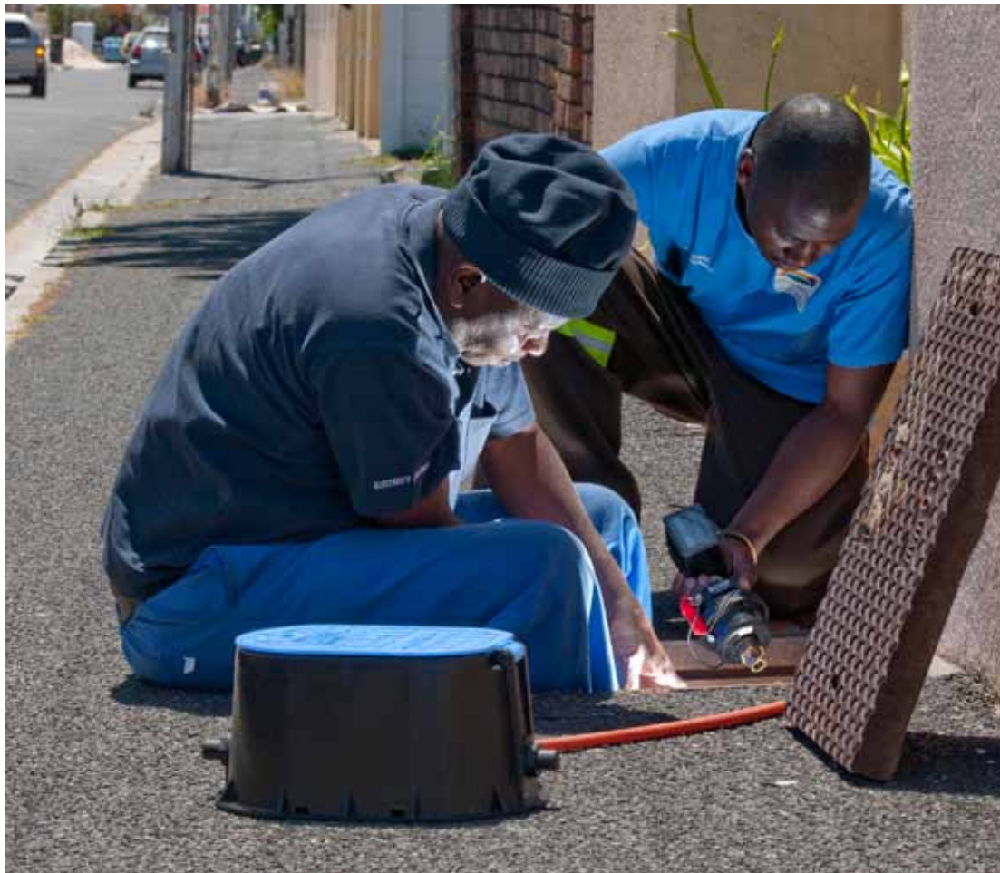
Part of the City's water demand management programme includes the installation of water management devices.
