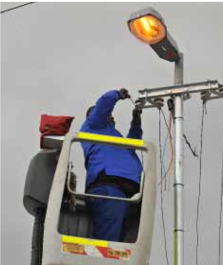
The refurbishing and maintenance of electricity infrastructure will continue.
