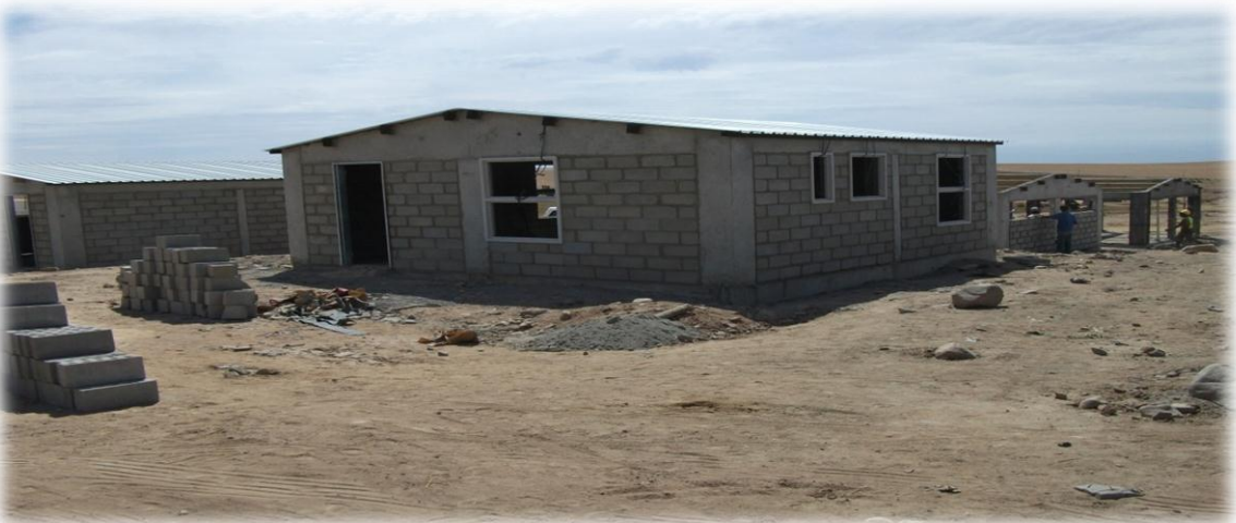
New houses being constructed at Piketberg
