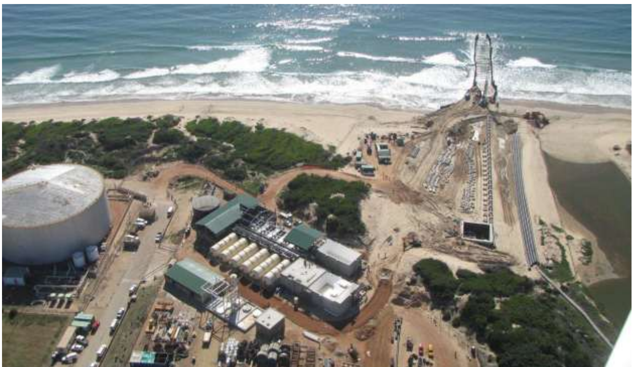
Mossel Bay 15ML Desalination Plant under construction
