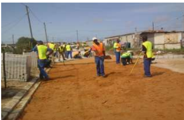
EPWP, Paving of Barnard Street
