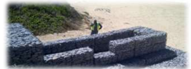
Upgrade Stormwater Outlet Outeniqua Beach
