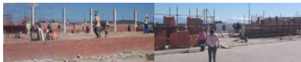
Thusong Centre under Construction: Estimated project completion date June 2013
