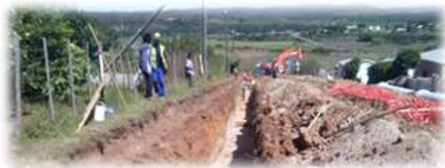
Brandwacht: Upgrading of Streets and Stormwater
