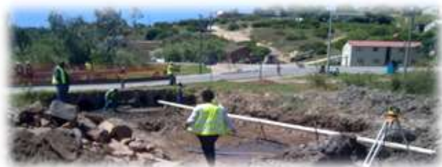
Greenhaven: Upgrade Stormwater Drainage Gelderbloem Street
