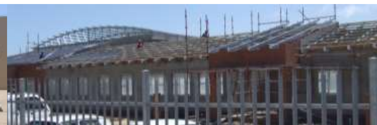
Thusong Centre Under Construction
