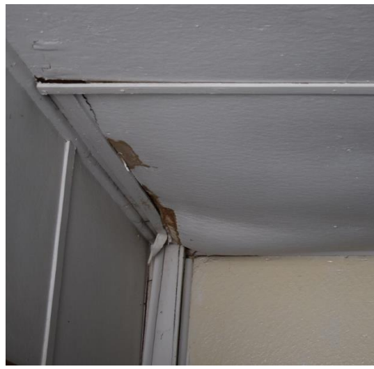
Image 8: Damage to the ceiling caused by water leaks
