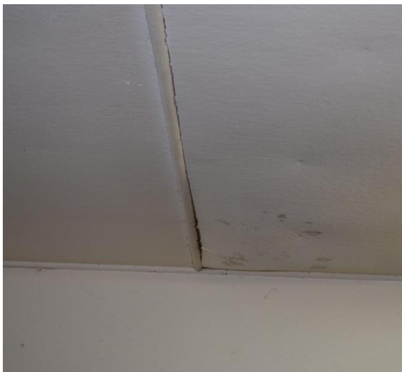
Image 8: Damage to the ceiling caused by water leaks
