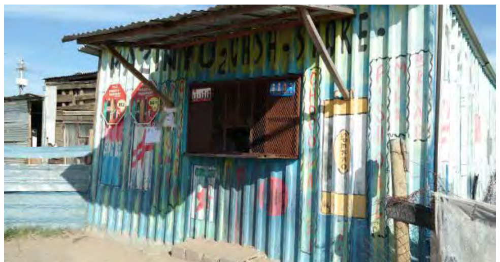
Structure used as spaza shop
