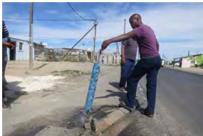
Running water tap in Kosovo
