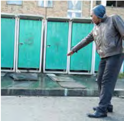
Flooding around toilet block in Gxagxa
