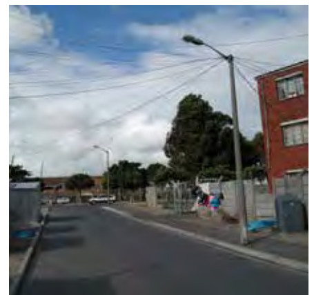
Electrical connections in GxaGxa
