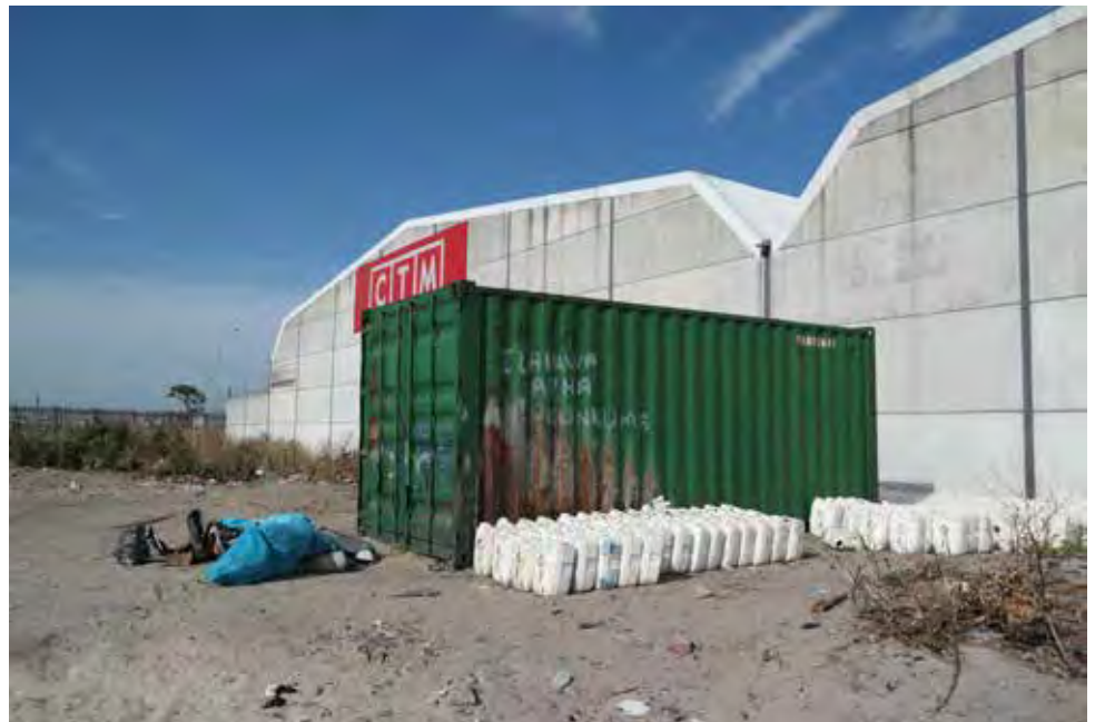
Waste removal area with portable toilets
