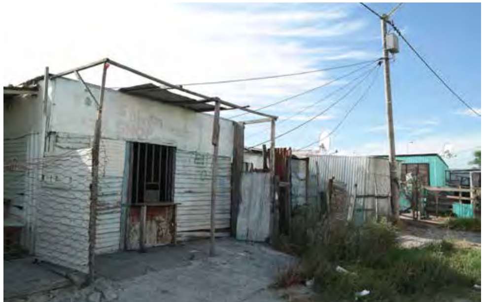
A structure is used as a spaza shop
