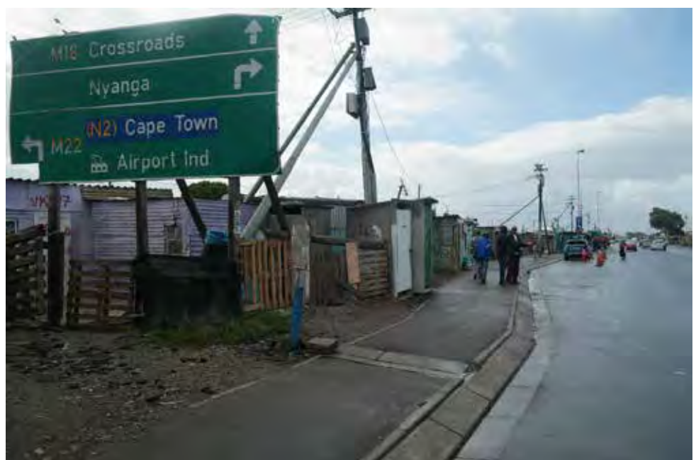
Proximity of Vukuzenzele to the airport
