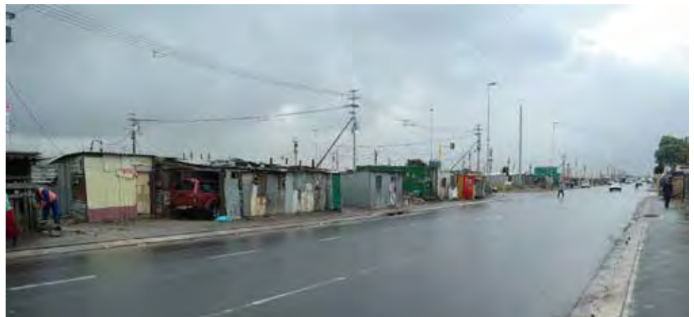
View of electrical connections in Vukuzenzele
