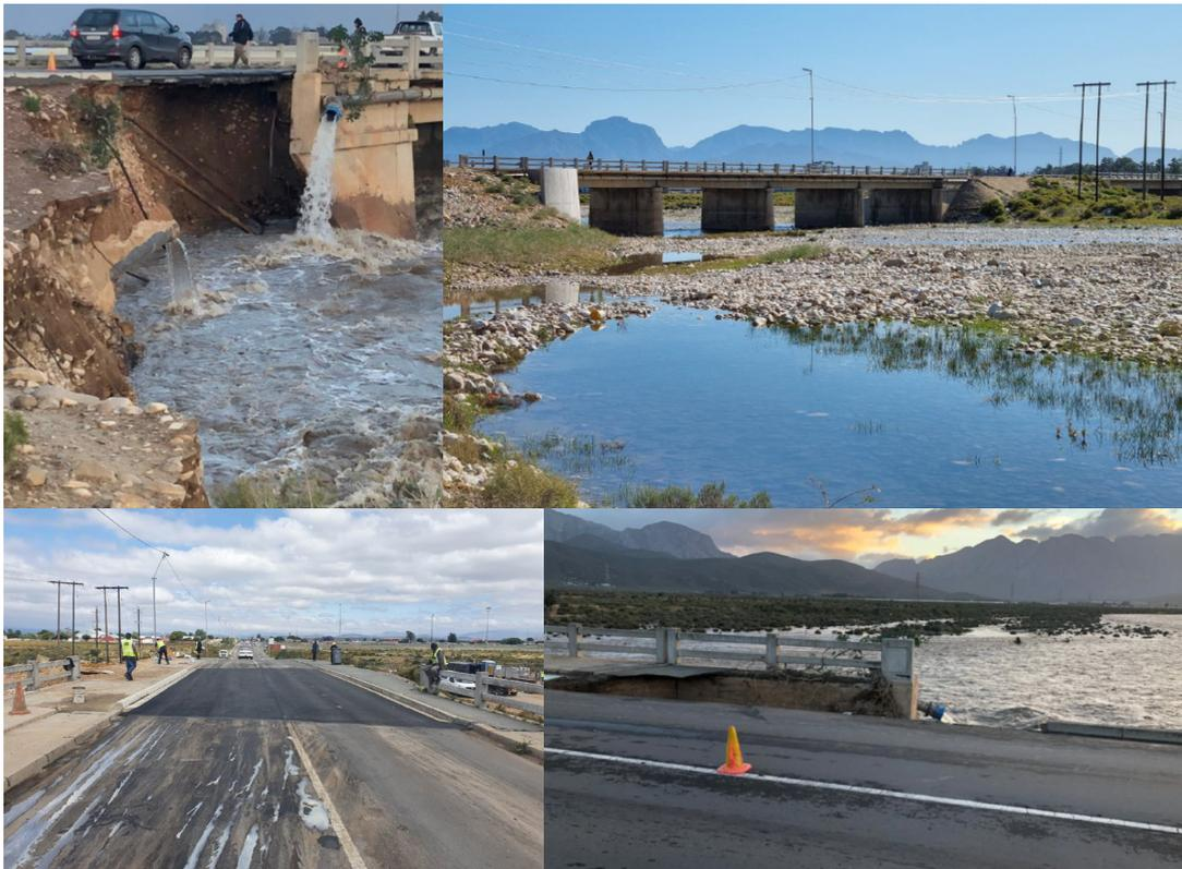
**Figure 77:** Damaged and repaired Zwelethemba bridge, Breede Valley Municipality
