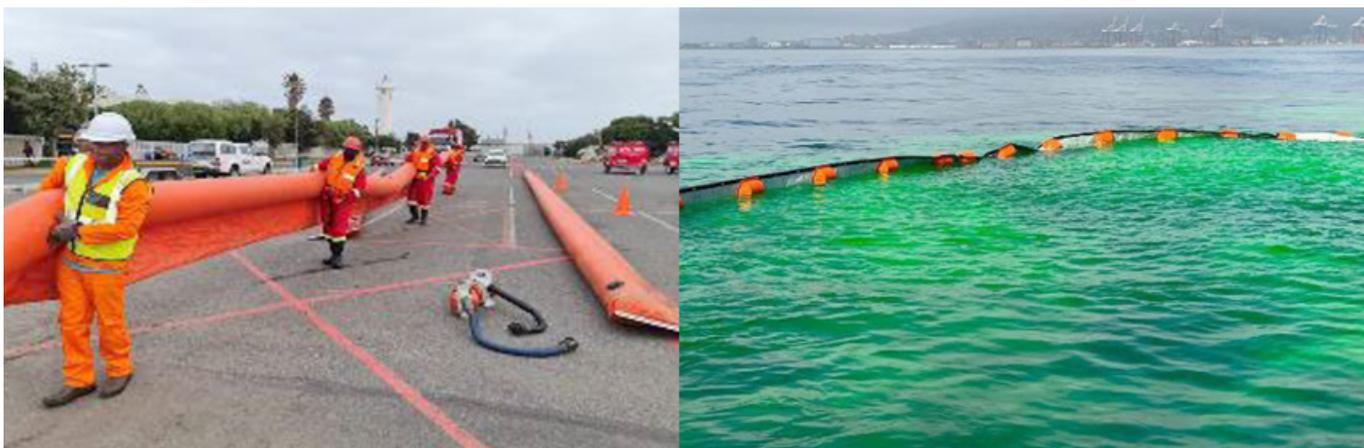
**Figure 51:** Fence boom deployed
