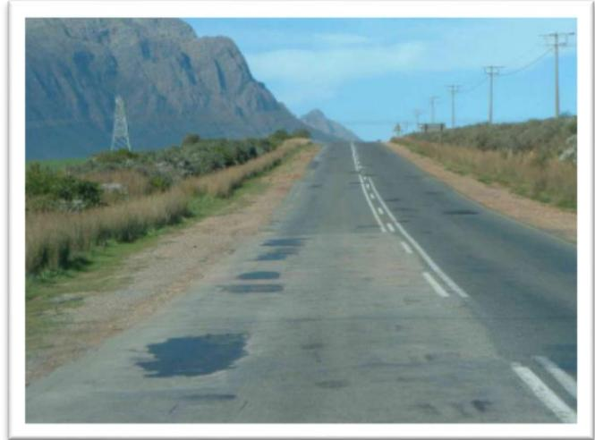
Picture 5-2: TR22/1 on 12/7/2007 showing development of potholes
