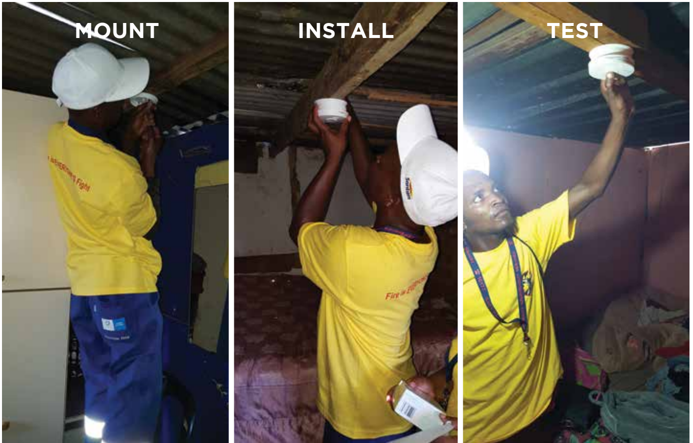
Figure 14: Installation of smoke alarms by the installation team
