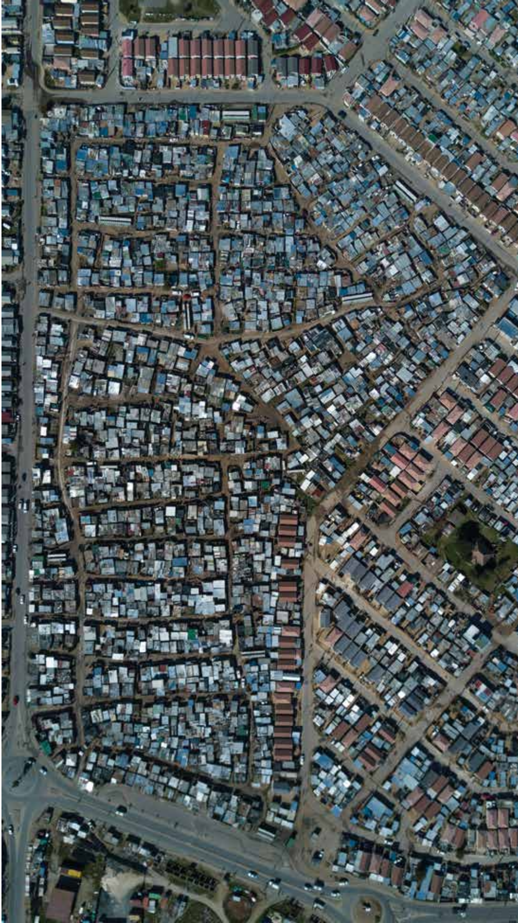
Figure 8: Aerial view of Wallacedene TRA in 2017s. (Source: Courtesy of Sullivan Photography, 2017)
