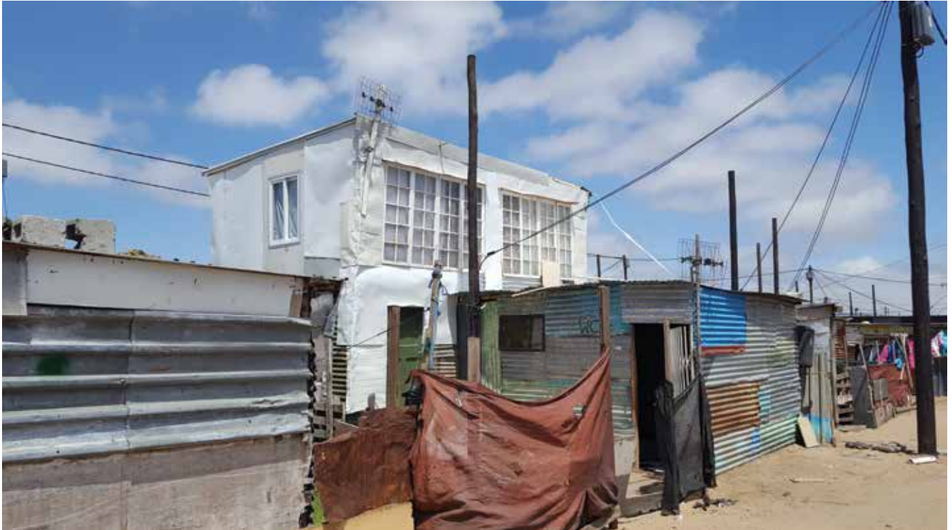
Figure 6: A variety of unregulated construction methods and materials are utilised with limited space both in and surrounding the structures
