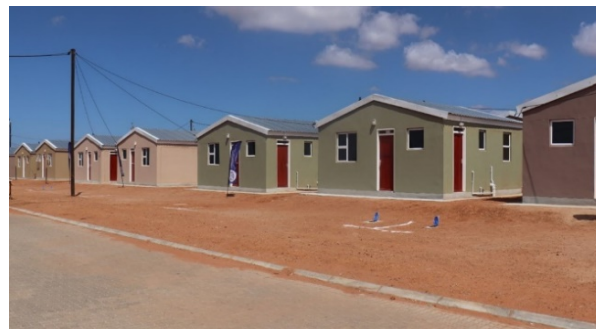
Lamberts Bay Housing Project (Cederberg Municipality)
