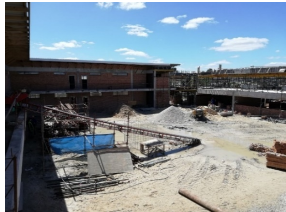
Umyezo Wama Apile High School (Theewaterskloof Municipality)
